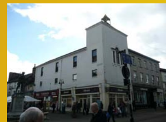
Shop front refurb, Kendal
