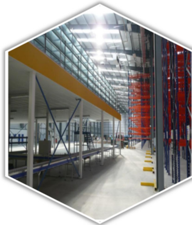
Pictured : main warehouse Before (left) & after (right).
