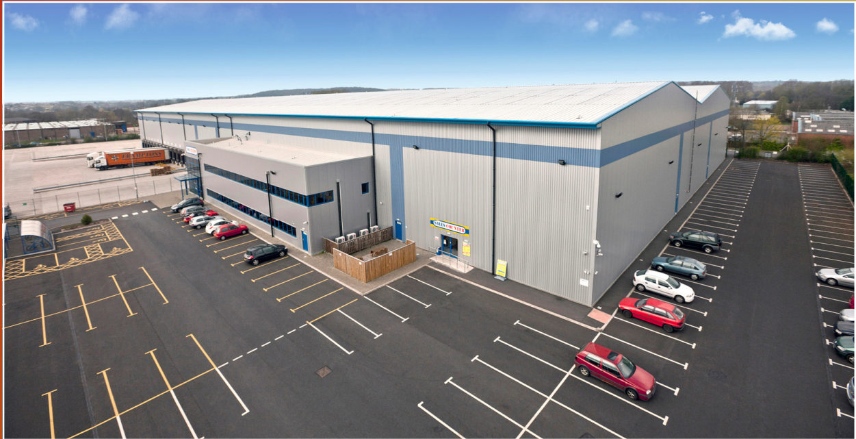
Above: Toolstation Redditch Distribution Centre and Trade Counter on Completion.
