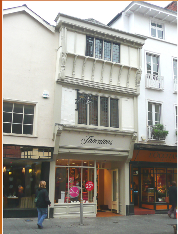
46 High Street, Exeter: complete (above), timber decay exposed (left) and conserved interior (below).
