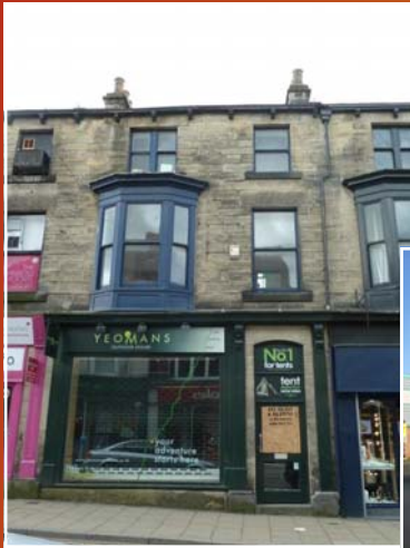
Smith Nicholas Harrogate and Castleford, before works commenced
