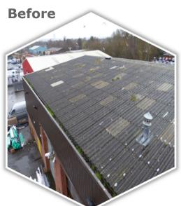
Bradley-Mason LLP were initially instructed to assess the existing asbestos cement profiled roof covering and to provide an options appraisal with associated budget costing.
