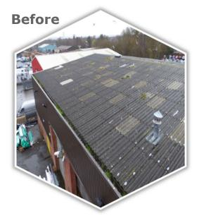
Bradley-Mason LLP were initially instructed to assess the existing asbestos cement profiled roof covering and to provide an options appraisal with associated budget costing.
