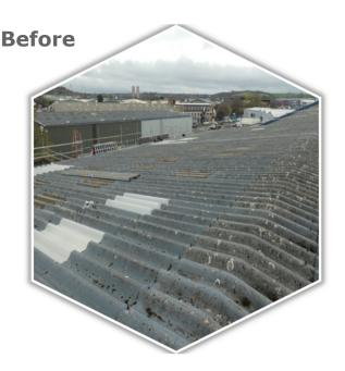
Bradley-Mason LLP were initially instructed to assess the existing asbestos cement profiled roof covering and to provide repair options appraisal with associated budget costing.
